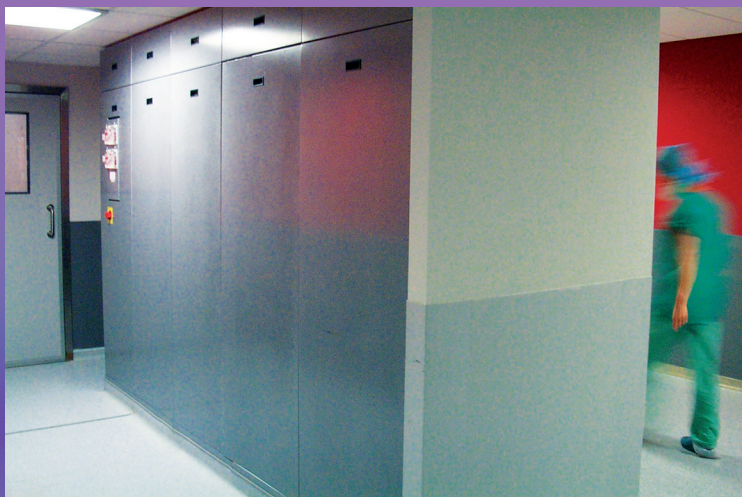
Technical closet for recovery room air treatment
